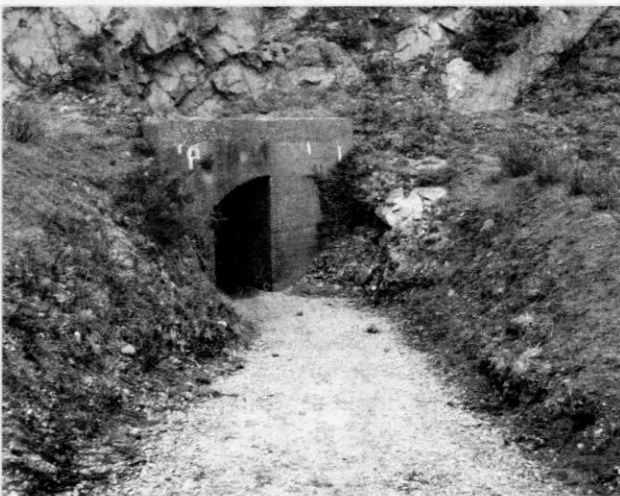
Laye Tunnel - Roadside entrance to Laye Tunnel
